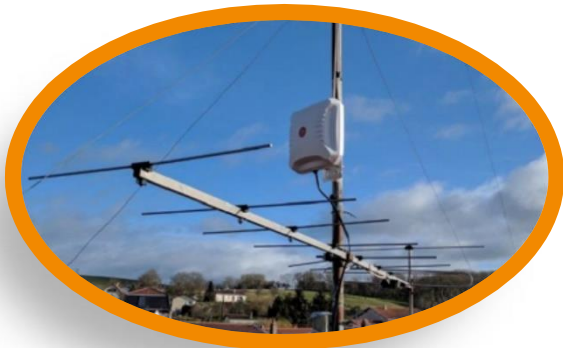
Figure 4. Poynting XPOL-2 Installation
