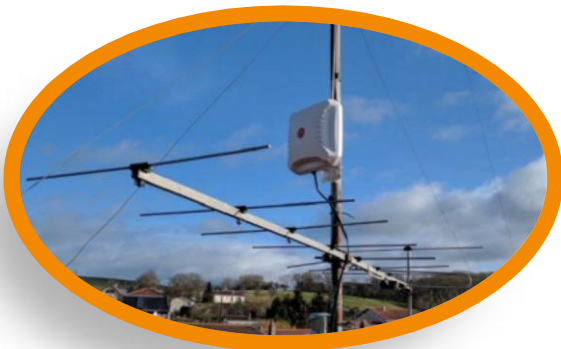
Abb. 4. Poynting XPOL-2 Installation
